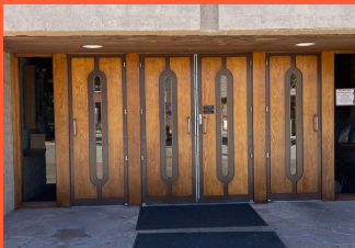
The wood around the stained glass was sanded, stained, and sealed inside and out.
